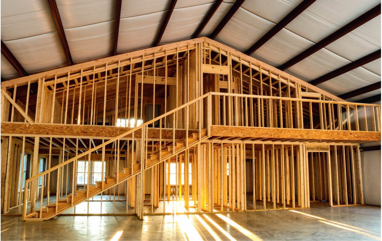
Interior barndo framing looks like a house within a house. This is one of the unique facets of barndominiums and allows for adaptability and structural integrity.
