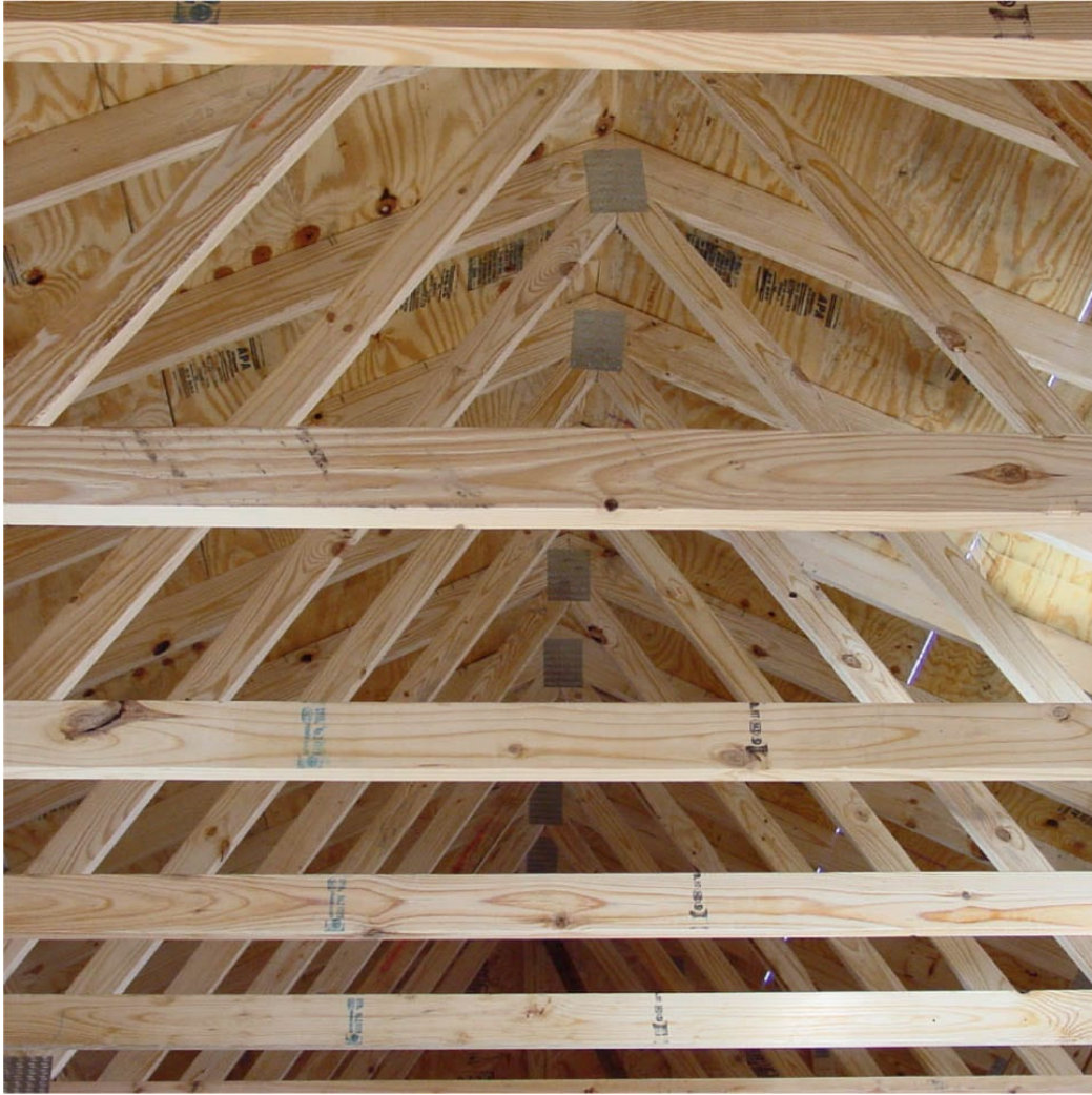
A completed wood-framed roof. Notice the prefab trusses, and the underside of the roof sheathing on which the final roof will be placed.
