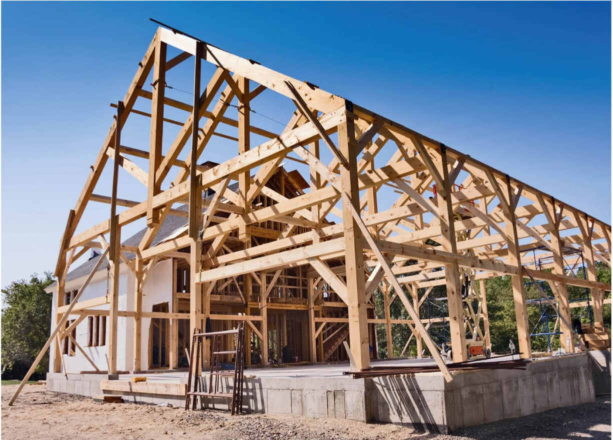
A post-and-beam barndo extension on an existing house awaits a steel roof and steel wall panels.
